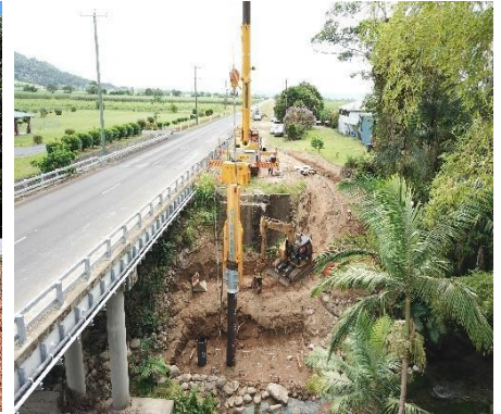
Josephine Creek Piling
