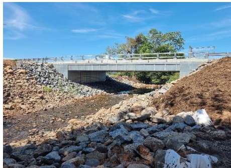
Rocky Creek Bridge
