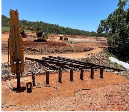
Rocky Creek Abutment Piling
