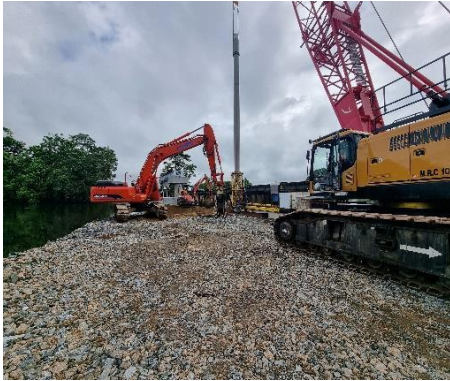
North Johnstone Piling
